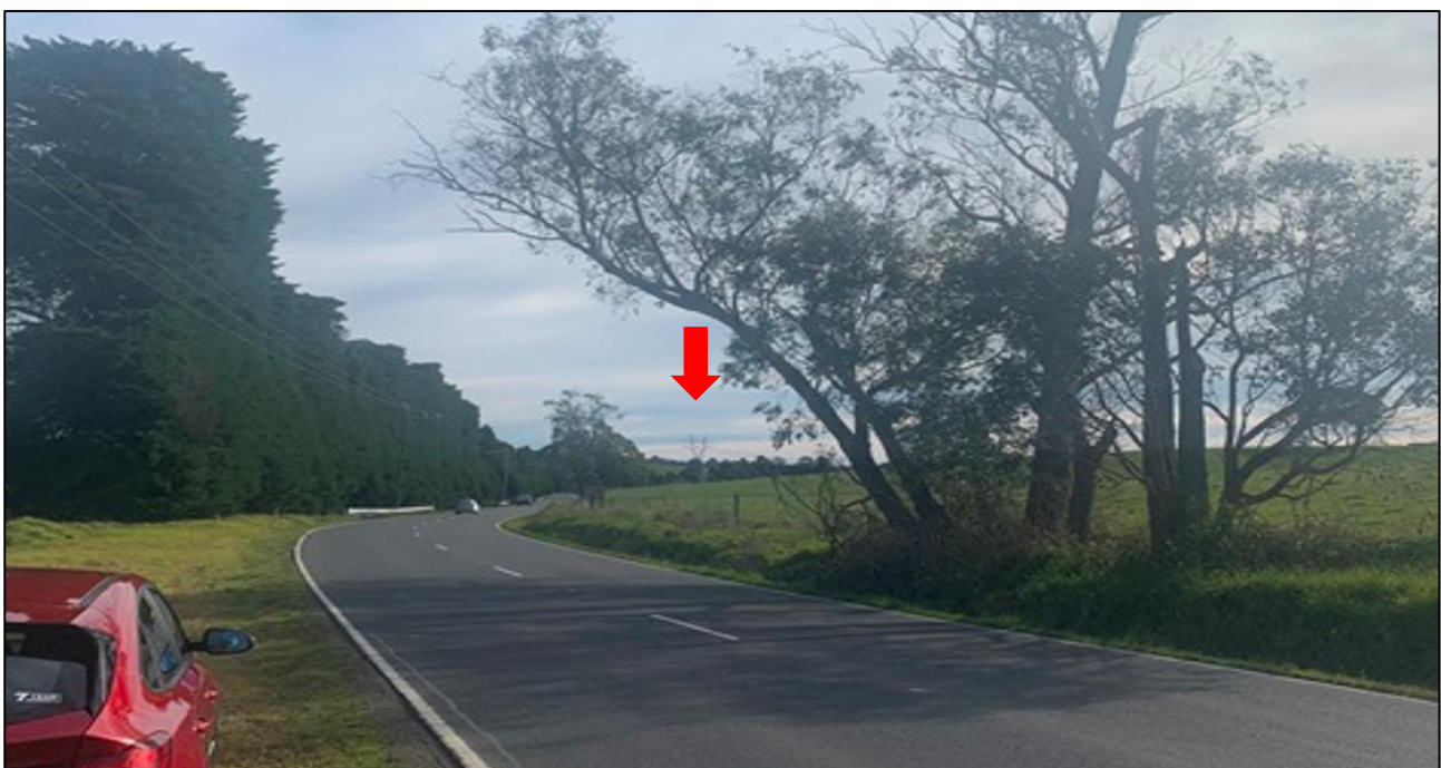
Figure 6: Existing high voltage towers in surrounding landscape (Field Investigation, 20 August 2022).
